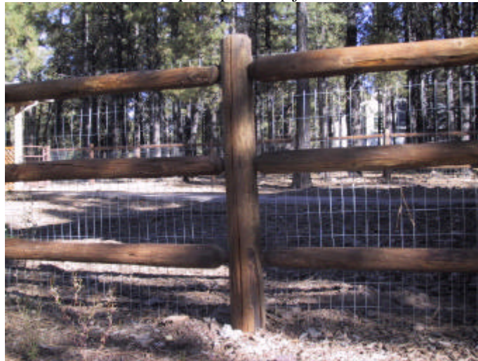
Sample split rail fence with interior fastened metal mesh.
